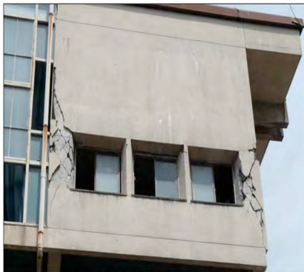
Typical 'short-column failure' in the upper floor of an old school building in Mito. This indicates strong shaking. (Source: Impact Forecasting)
